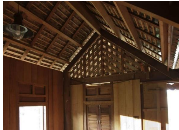
Figure 3.74. The gap between walls and roof (Author)
