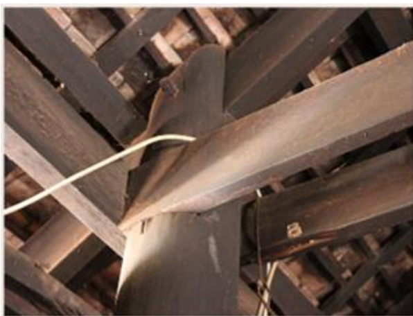
Figure 3.54. Roof & Column Joint Structure (Author)
