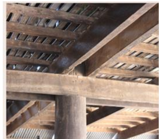
Figure 3.55. Floor & Column Joint Structure (Author)
